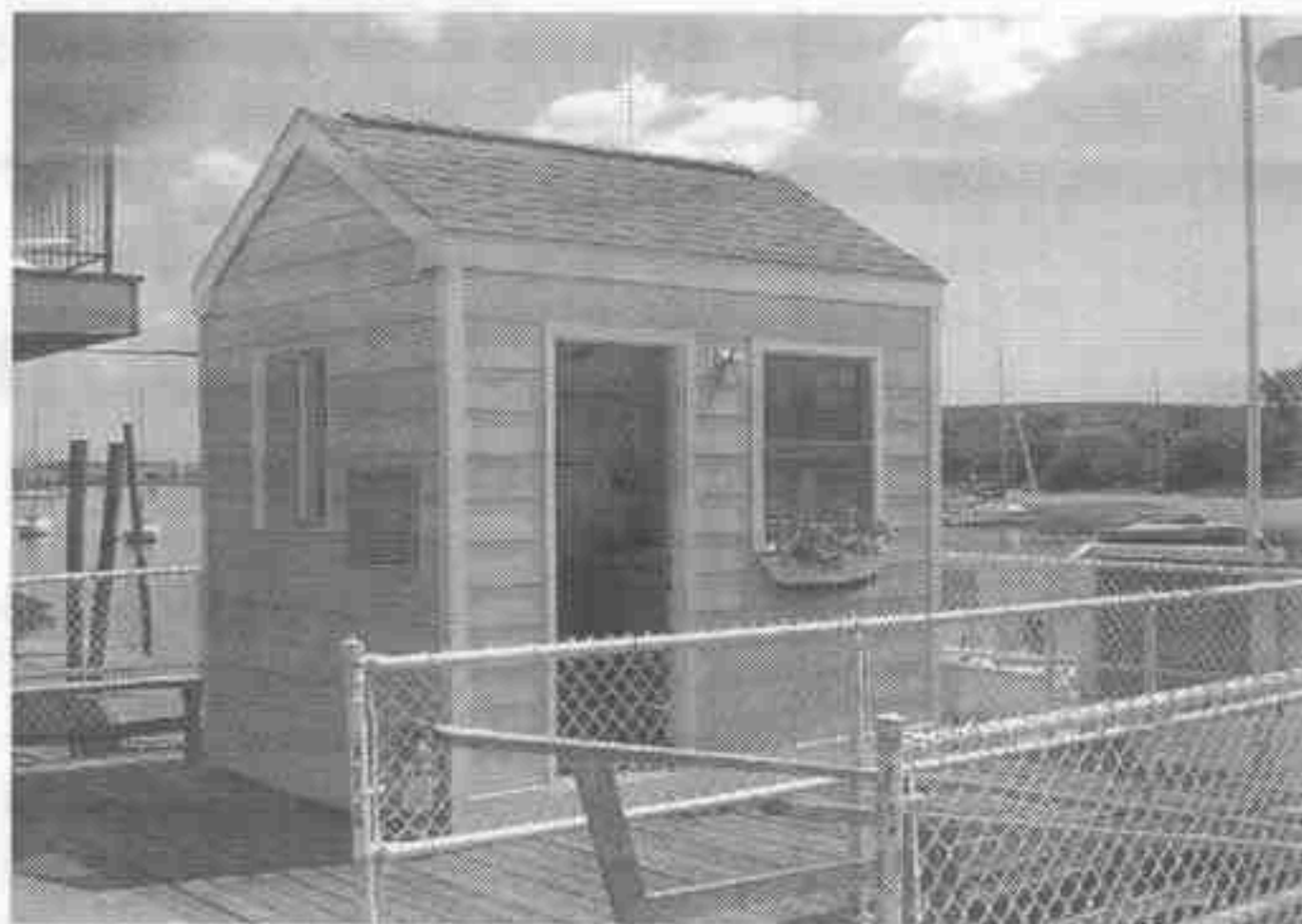
Pretty Picture. This building used by the dock personnel was constructed by members with materials donated by members. Some of the movers and the shakers involved are; Gerry Weiss, Builder; Chris Bilyard, Henry and Gerety, material donations and George Nemeth, Clearview Glass, material donations, and many other members, sorry to any I missed.
